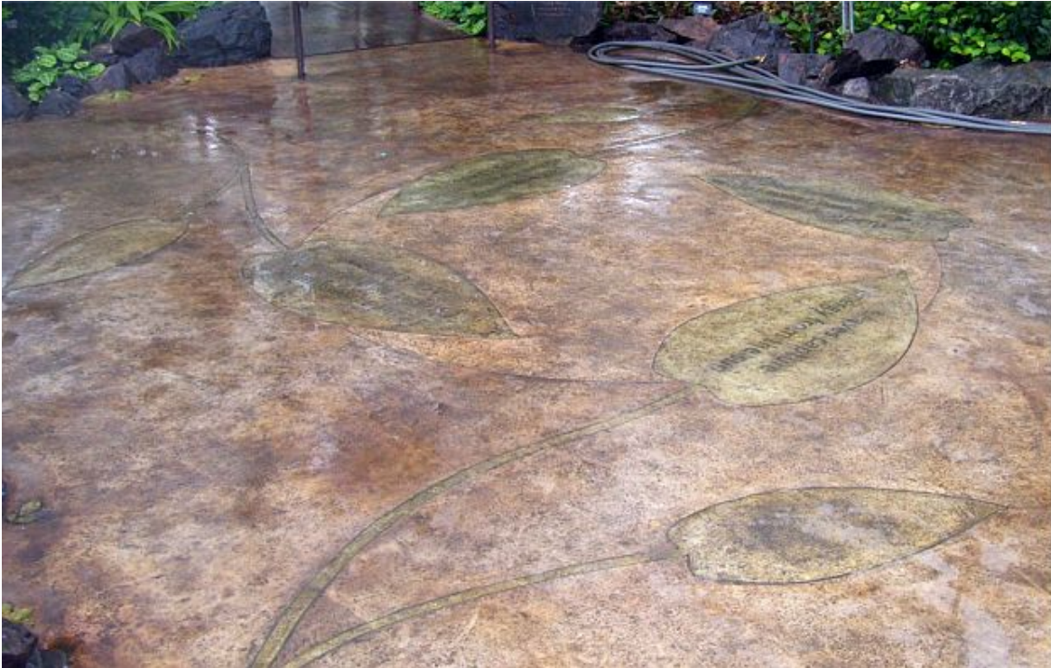
Figure B-19. Central Plaza , where four leaf-shaped Synthesis labels were embedded in the concrete floor.
