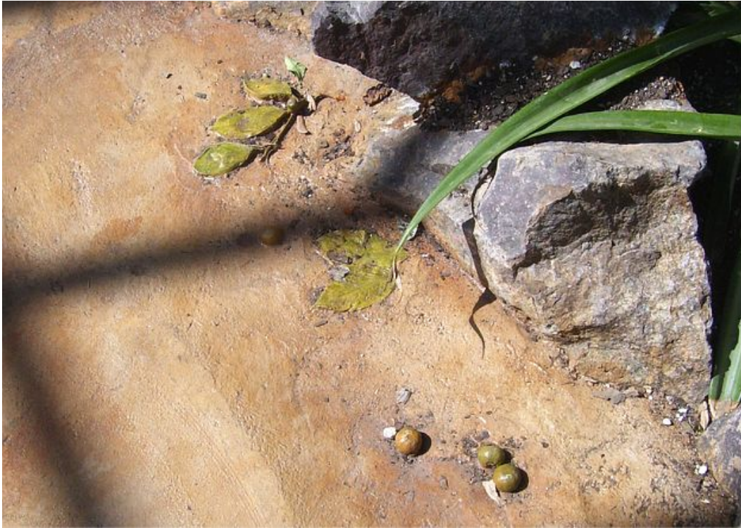
Figure B-21. Artificial fruits and leaves included as part of the concrete floor.
