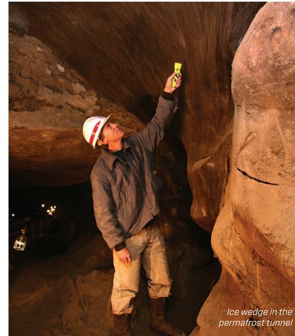
Ice wedge in the permafrost tunnel
