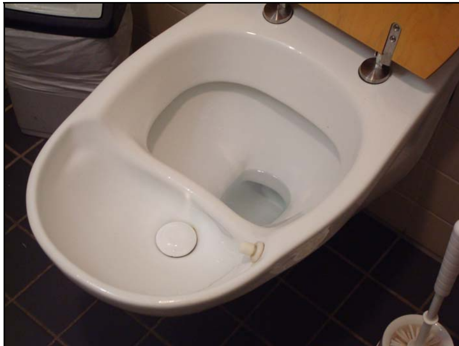
Figure 31: Source separation of waste at Universeum, Gothenburg.
