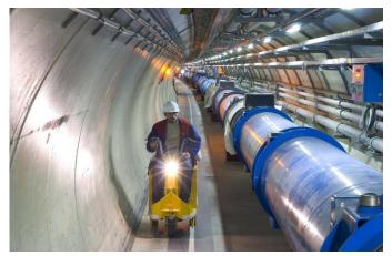
Moderator's verbal description for second photo: Just to give you a sense of scale, here's a photo of part of the tunnel. The Large Hadron Collider was built to study the universe's tiniest particles. You learned in school about particles like protons and neutrons, but there are many many other much tinier particles that scientists study. In the tunnels, beams of particles are accelerated to almost the speed of light and guided in opposite
